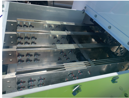
Internal Trough Bus Connection 4000A Trough is certified UL 870
